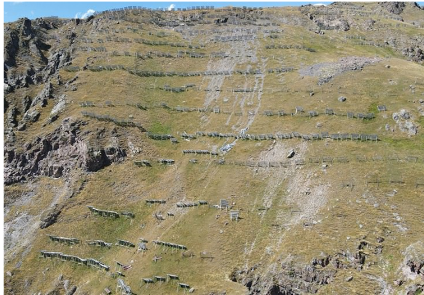
Figure 7. Snow retention structures on the southern slope of Mount Elbrus. Photo August 2022.
