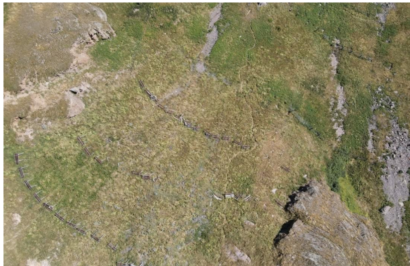
Figure 8. Destroyed sections of snow retention structures on the southern slope of Mount Elbrus. Photo August 2022.
