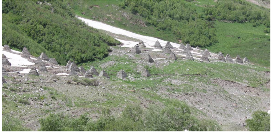
Figure 4. Avalanche-braking structures on the northern slope of Mount Cheget. Photo, June 2022.
